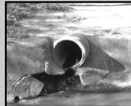
**Culvert:** A pipe of any size that diverts water such as a stream to flow under a roadway or other land.
