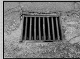
**Drain Manhole:** A covered opening in a street which provides access for cleaning and repairing of a stormwater system. *(Typically connecting two other stormwater drainage structures)*
